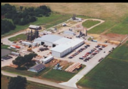
UOP Callidus 82,000 sq. ft. manufacturing and fabrication facility in USA
