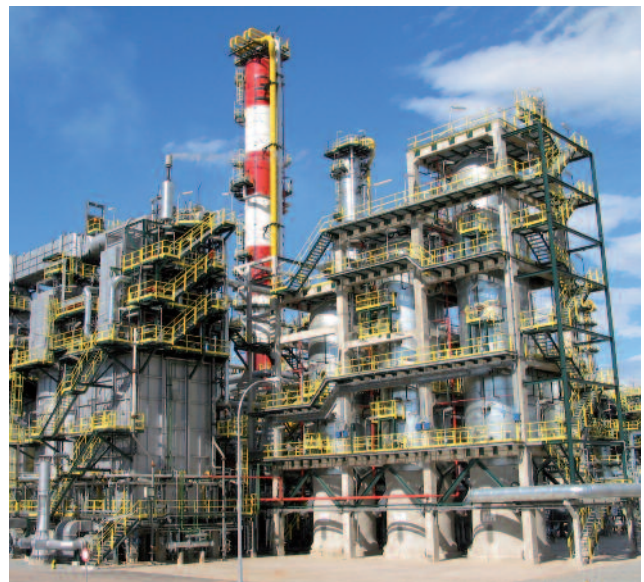
Single-stage once-through hydrocracker
