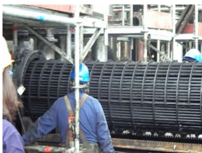
Bottom exchanger extraction
