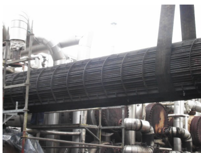
Bottom bundle as extracted for visual inspection
