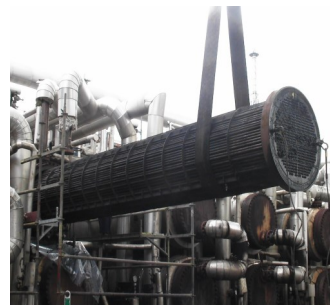
Bottom bundle as extracted for visual inspection
