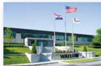
1995 Watlow headquarters following two expansions
