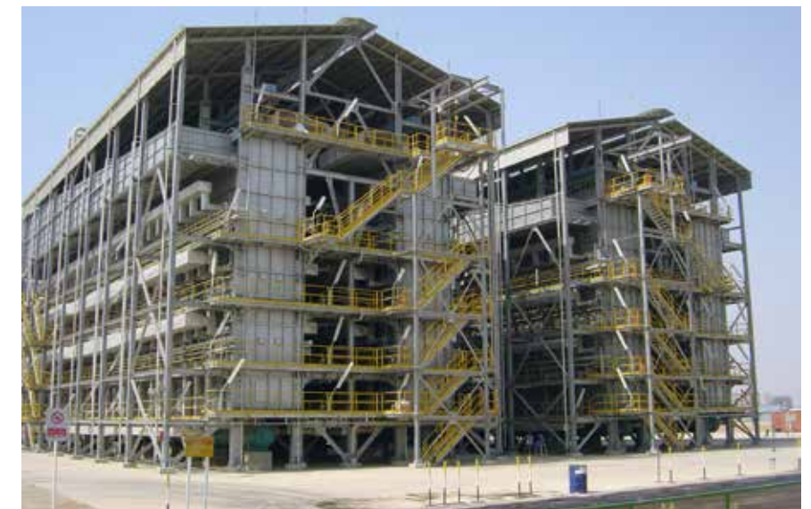
More than 250 Topsoe radiant wall steam reformers are operational today
