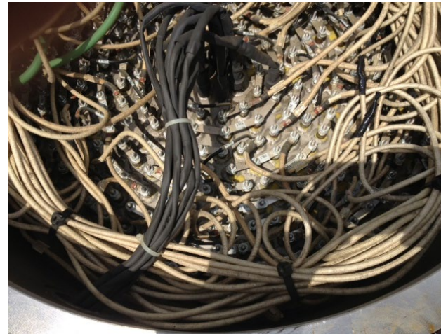
~1 MW Low Voltage Heater (460V)
