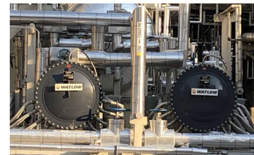
Heaters for Acrylic Acid process, LG Korea
