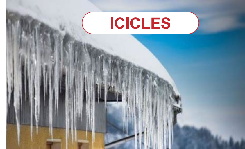
FROZEN WATER PIPES
