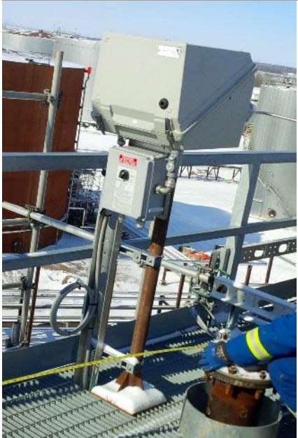
Instrument winterization / tubing bundles
