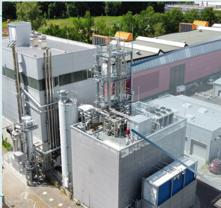
HTW® Facility at TU Darmstadt (Germany) (Energy Systems and Technology)
