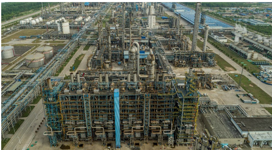
Wuhan 800/1,100 KTA Ethylene Complex
