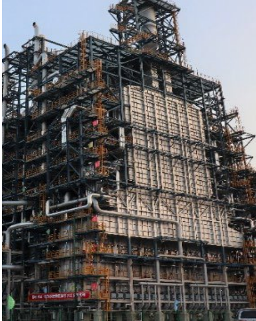
Zhenhai 150 KTA Single Firebox Liquid Feed Furnace
