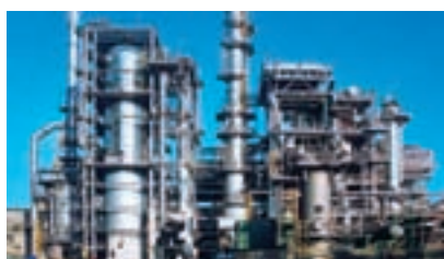
Middle Distillate Desulphurisation Unit for Shell Deutschland Oil GmbH in Wesseling, Germany
