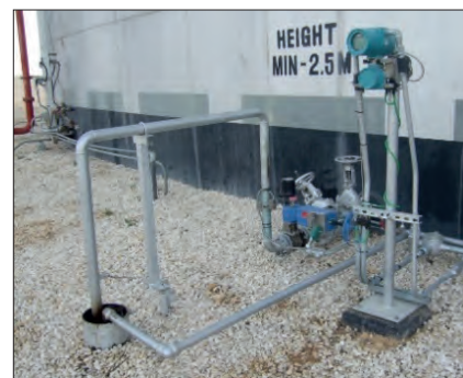
Figure 4 Sound velocity dewatering system set-up
