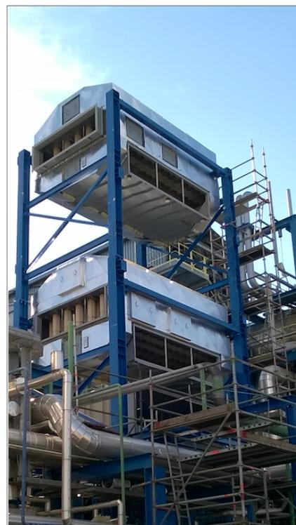
**Figure 6** HeatMatrix air preheater in a fired heater
